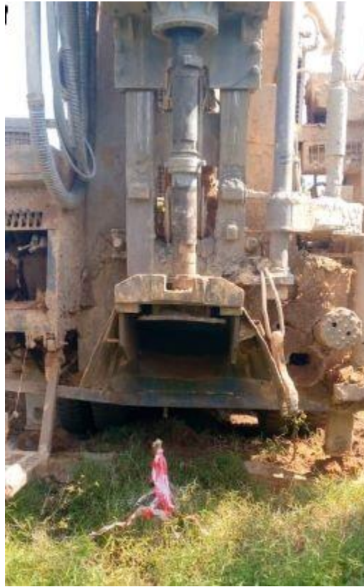
Picture showing rig positioned at recommended VES point
