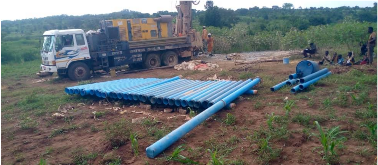
In the above pictures; PVC casing pipes aligned for installation process.
